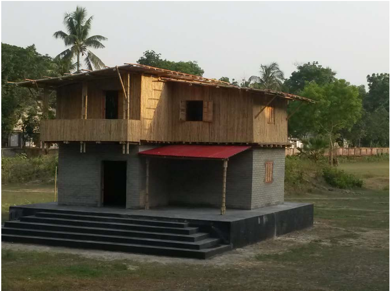
Figure 1 A clinic in rural Bangladesh built with Earth, Bamboo and Jute
